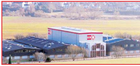
Headquarter of the IBC Wälzlager GmbH at the industrial area of Solms-Oberbiel
