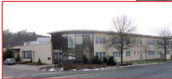
New plant in Asslar
